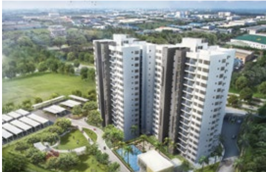
The Habitat Binh Duong residential development is currently under construction at our first VSIP project. It will cater to the needs of professionals working in the province
