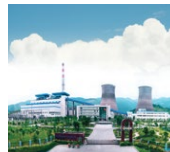
Formed a joint venture for a 1,620-megawatt coal-fired power project in Chongqing, China. The project's strategic mine-mouth location allows for power generation at a competitive cost
