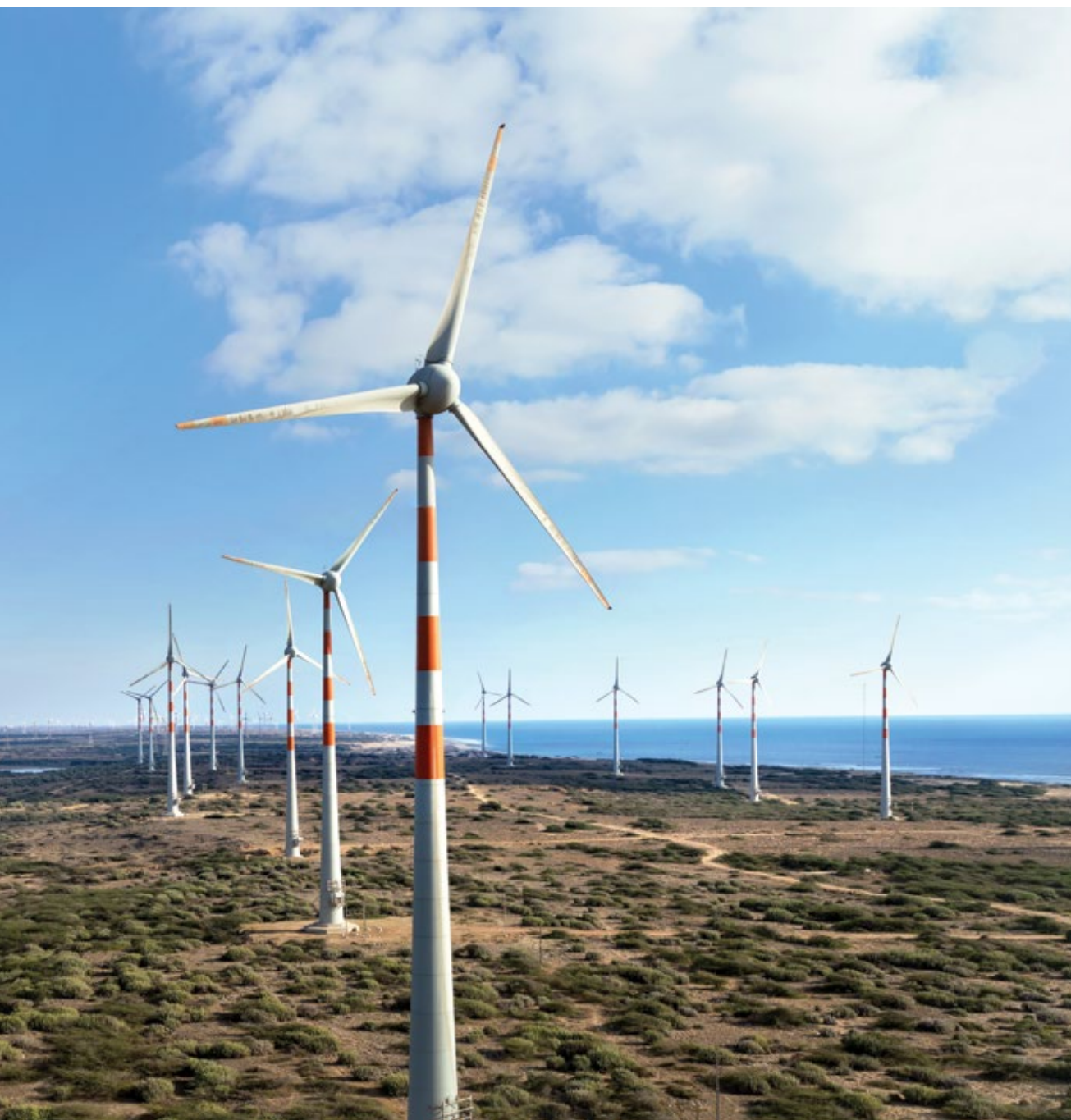
Sembcorp's wind power assets in Gujarat, India
