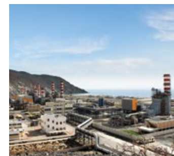
Successfully expanded desalination capacity at the Fujairah 1 independent water and power plant in the UAE to 130 million imperial gallons per day, making it one of the largest reverse osmosis desalination plants in the Middle East
